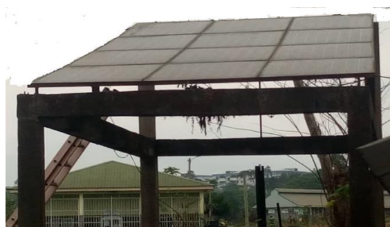
Fig. 13. Installed PV System
